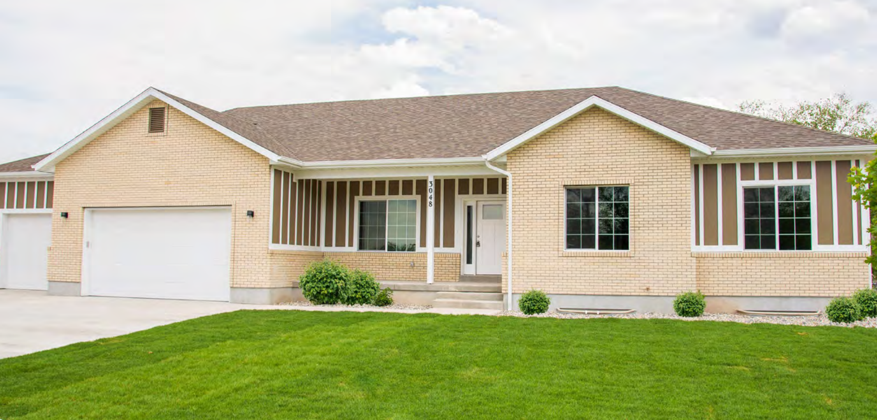
SLCC's most recent Project House located at Sunrise Pointe Court in West Valley City.
