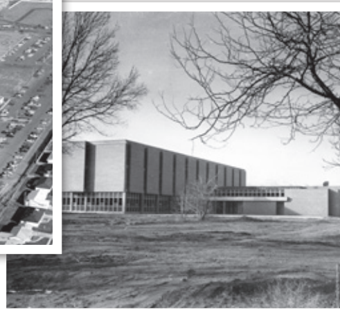
Nearly completed Nelson Administration Building, circa 1966.
